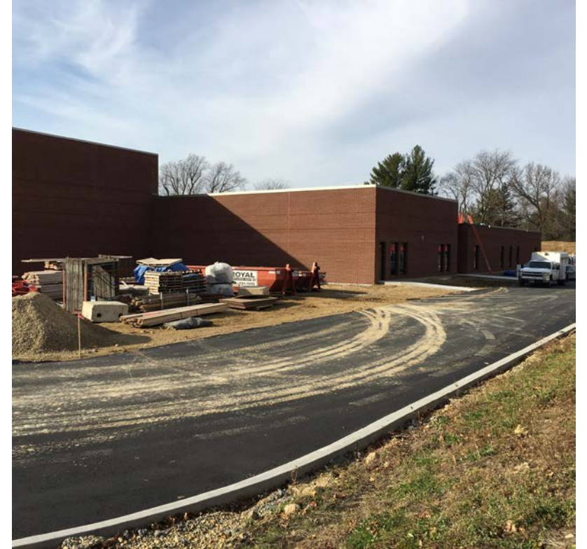
Exterior of building addition is mostly complete
