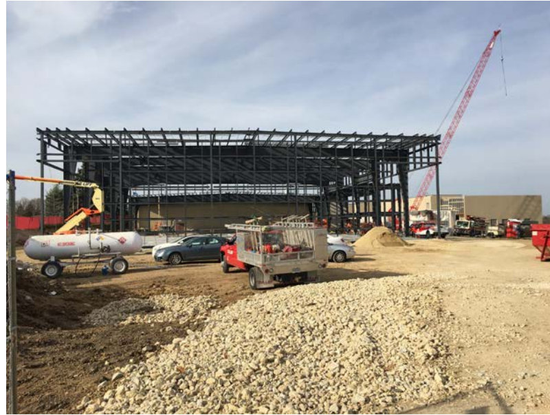
Gym and Pool progress
