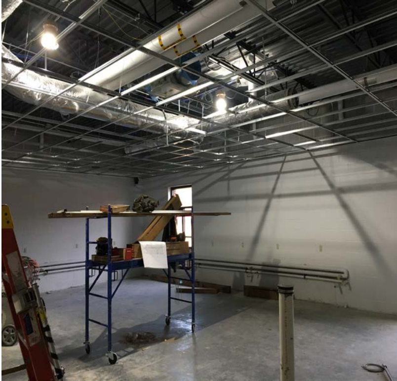
Ceiling grid installation has begun
