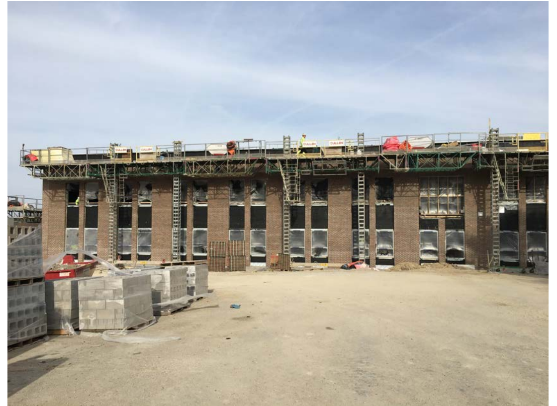
STEM addition progress – last of brick installation
