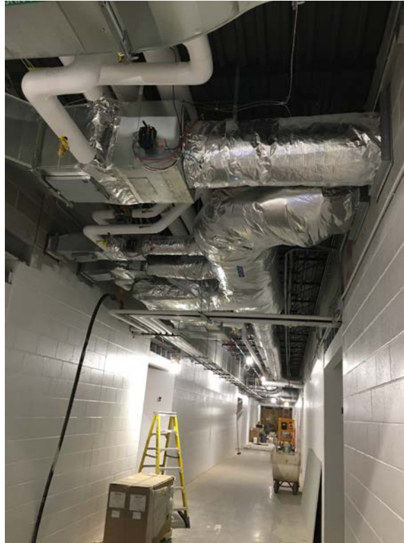
Mechanical installation is well underway
