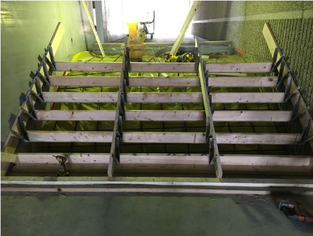
Stairs by pool – formed and ready for concrete
