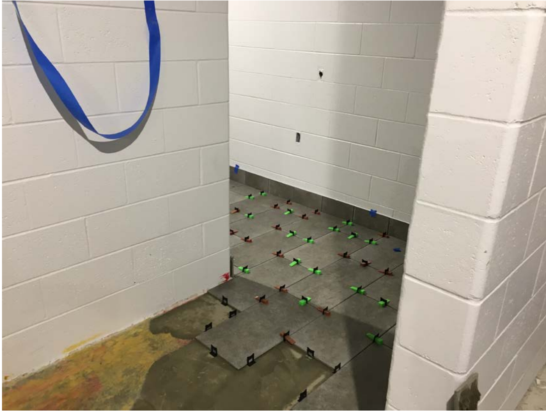
New bathroom tile being installed
