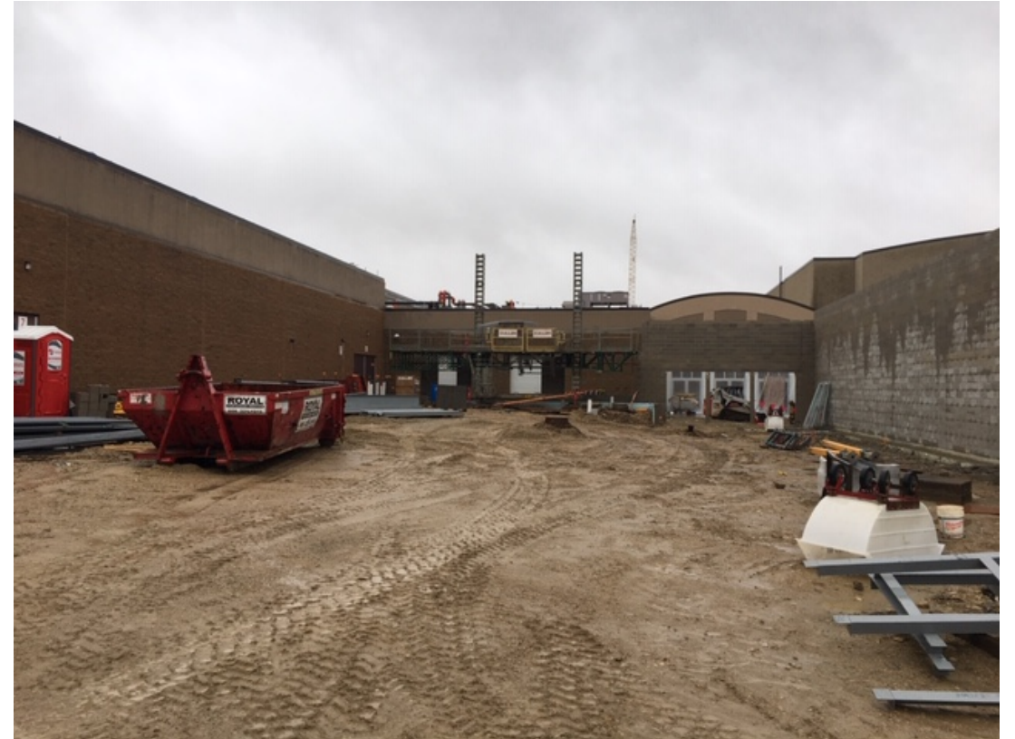
New connection corridor
