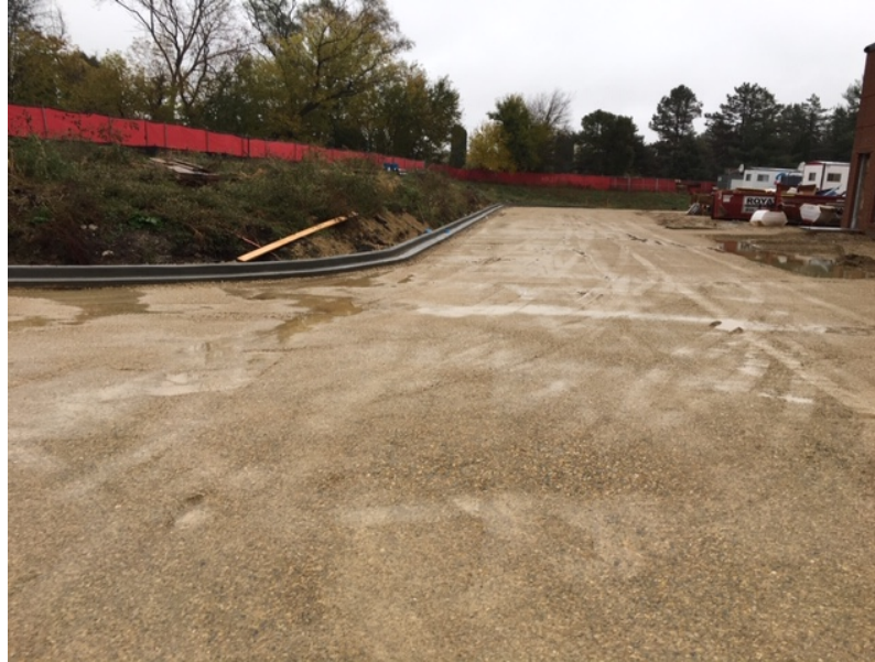
Driveway is ready for asphalt
