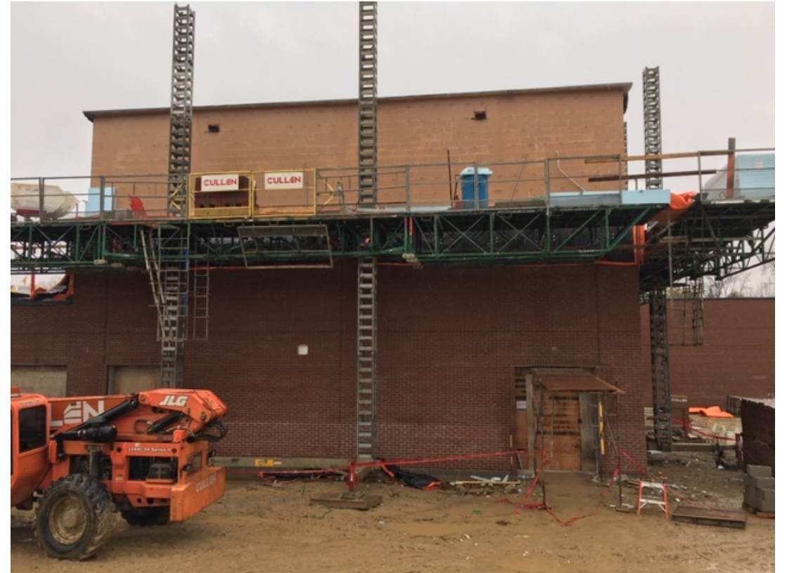
Last section of brick to be installed
