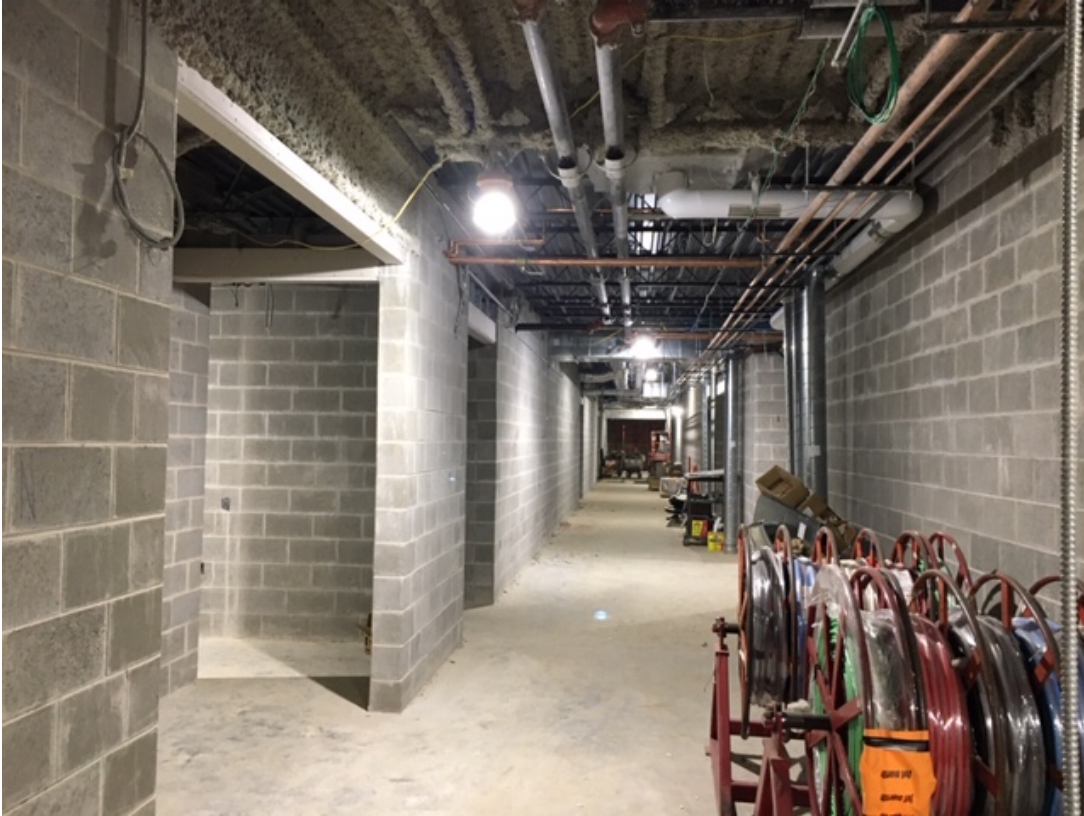
Corridor of the addition
