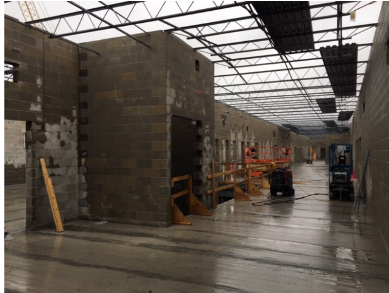
2 nd floor of STEM addition in corridor by elevator
