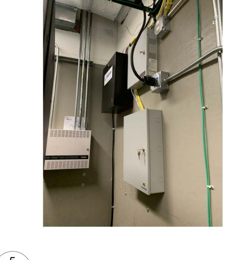
EXISTING KEYLESS ENTRY SYSTEM HEAD END E200 SCALE: NTS
